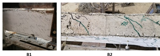
Figure 8. The Difference of the Cracks' Width Between B1 and B2 Beams.
