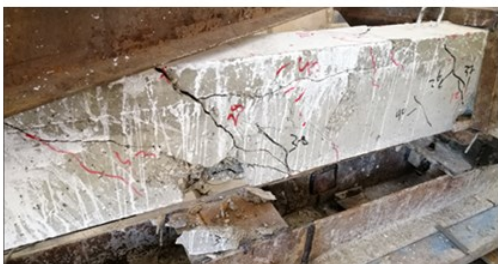
Figure 15. The Failure Pattern of BN Beam, Experimentally and Analytically
