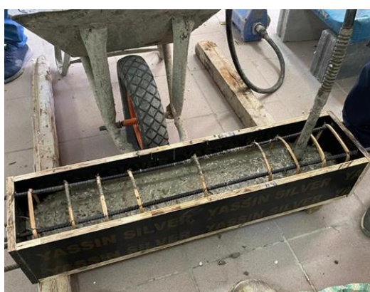
Figure 1. Vibration of concrete inside the molds.
